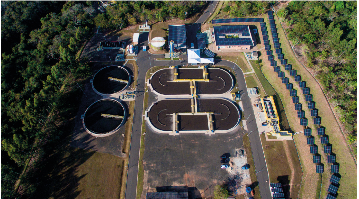
Solar energy at EDAR Mogi Mirim (Brazil)
